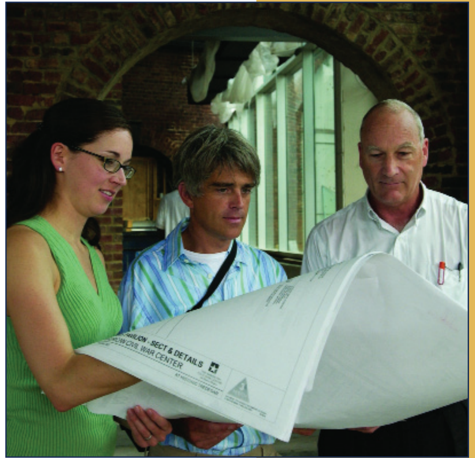
Jill Nolt, Todd Dykshorn, and Sanford Bond compare the plans to the work in progress.
